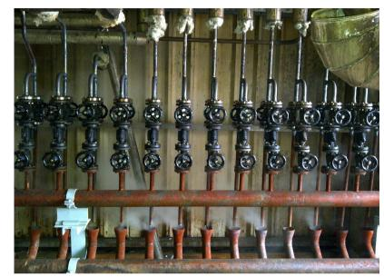
A chemical plant operator in Austria using the KLINGER KVN piston valve in a condensate collector produces phthalic anhydride. This process requires an immense amount of steam. In order to shut-off or by-pass the existing steam traps for maintenance the operator was looking for a safe and cost effective solution over the complete life cycle of the used shut-off valve.
